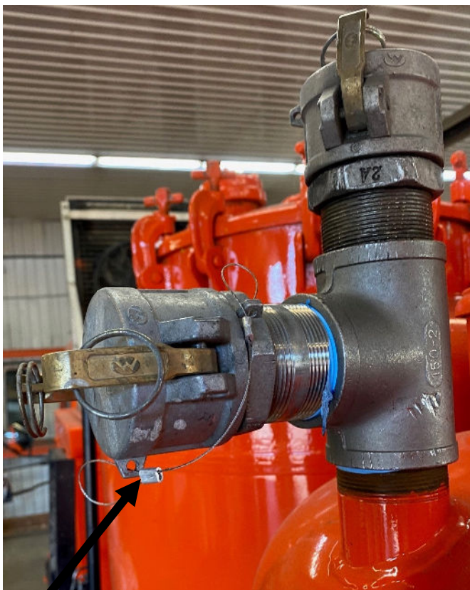
Wire Lanyard securing the cam-lock cap.
